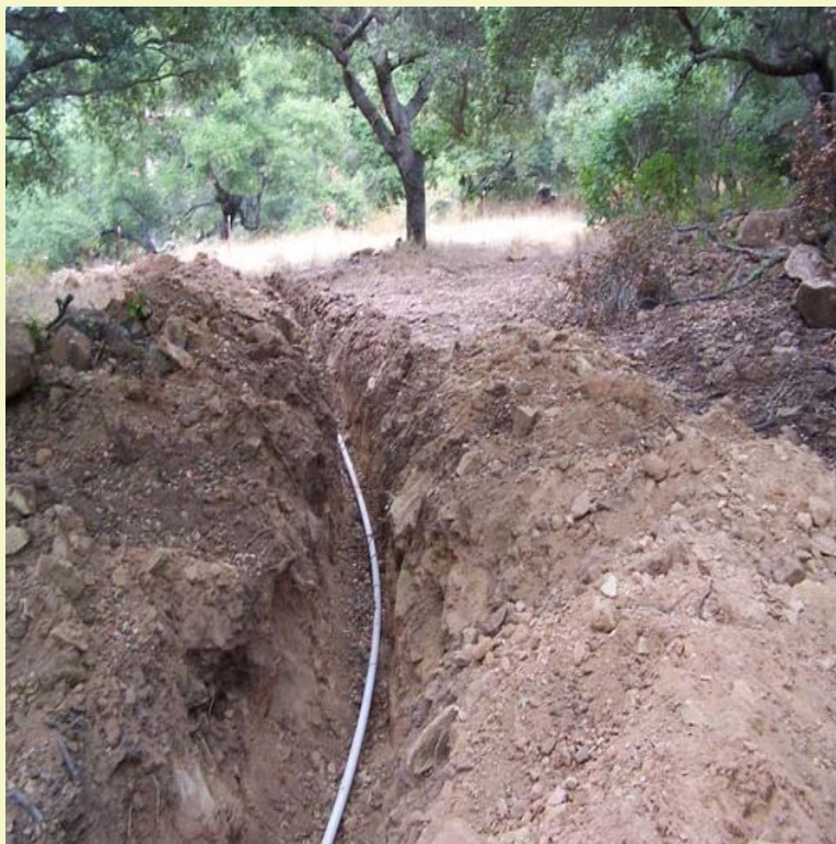
Stockwater pipeline installation
