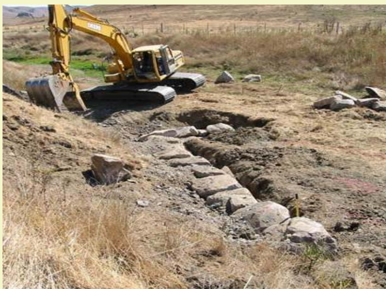
Rock J-hook under construction
