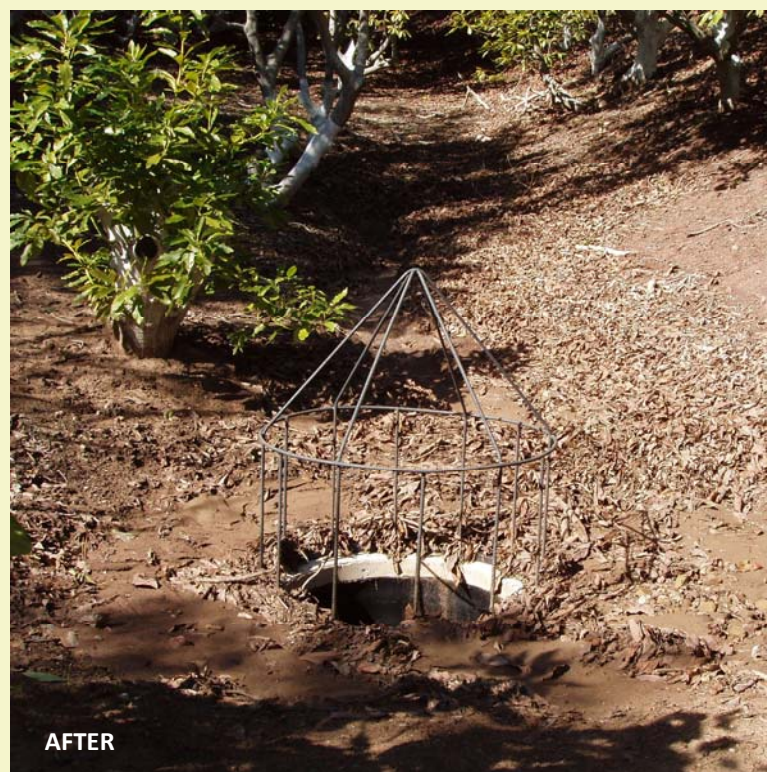
Combination of underground outlet, pipe drop inlet, and mulch used to safely carry water to a stable outlet
