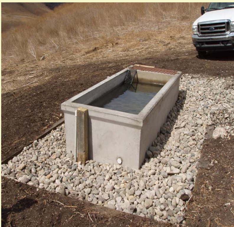
Stockwater trough installed on rangeland
