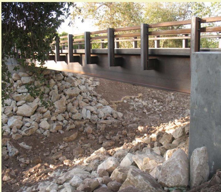
Low water crossing removed and replaced with bridge
