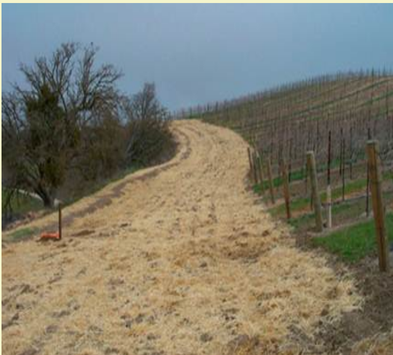
Critical Area Planting following construction of diversion and grassed waterway
