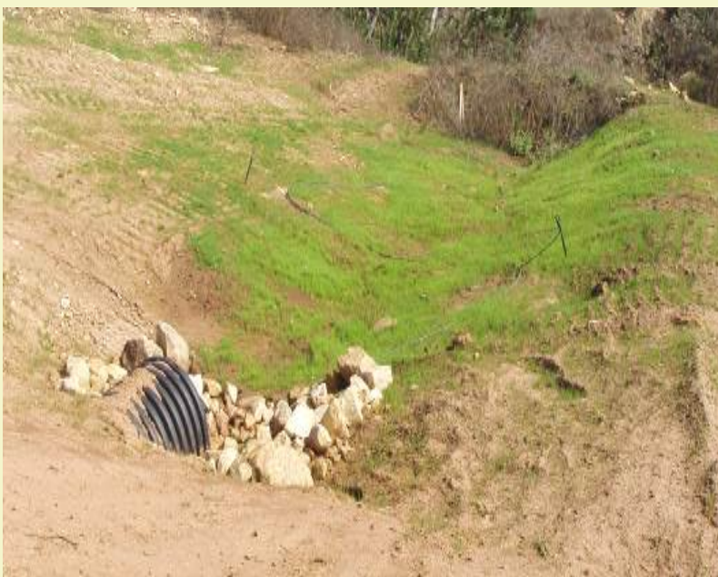
Critical Area Planting following construction of structure for water control
