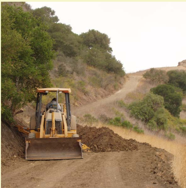
Regrading road to provide adequate surface drainage and prevent concentrated flow
