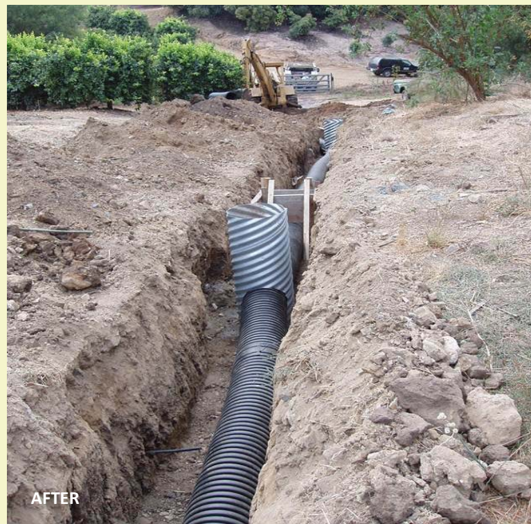
Installation of underground outlet and pipe drop inlets, used to safely carry stormwater runoff to a stable outlet
