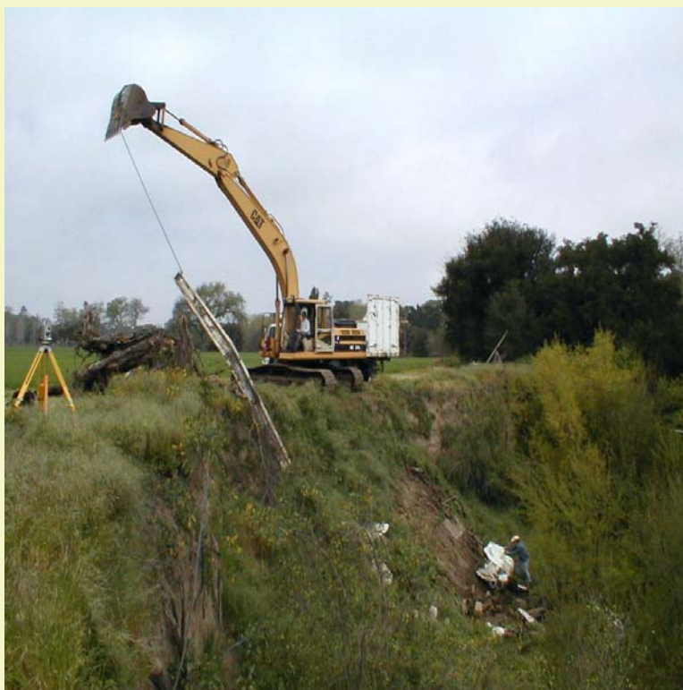
Crane removing trash from riparian corridor
